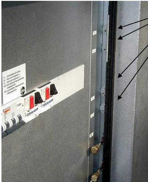
The spigots are positioned in pairs. The upper output measures pressure loss over the condenser/evaporator on the air intake side, while the lower output measures pressure loss over the condenser/evaporator on the extract air
