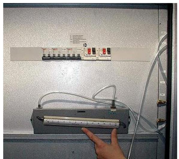
11. Measure fan motor power consumption. This must not exceed the power consumption value (see label).
